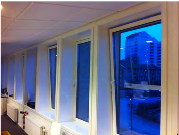
Figure 6. Images from the full scale test room. All 9 windows along the façade could be opened, i.e. tilted inwards individually, for a controlled change in the scattering properties of this boundary. In the opposite wall, all doors were closed when the effect of scattering was tested.
